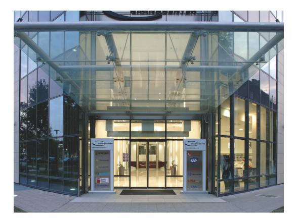
Automatic linear sliding door system with burglar resistance in accordance with resistance class RC2
